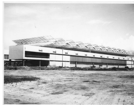
International Trade Fair, Accra, 1967, Pavilion A. GNCC, Vic Adegbite (chief architect), Jacek Chyrosz, Stanisław Rymaszewski (project architects). Private archive of Jacek Chyrosz, Warsaw (Poland).
